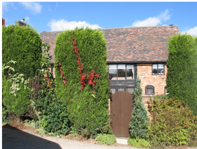
17 th -century timber-framed barn
