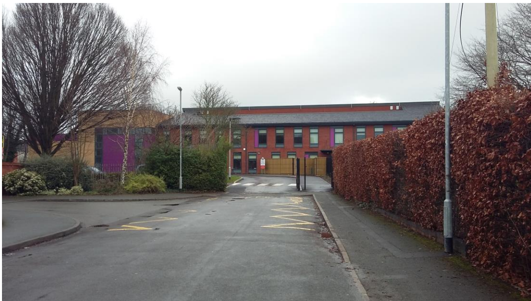
Figure 1: New two storey replacement building at Moorgate Primary School
