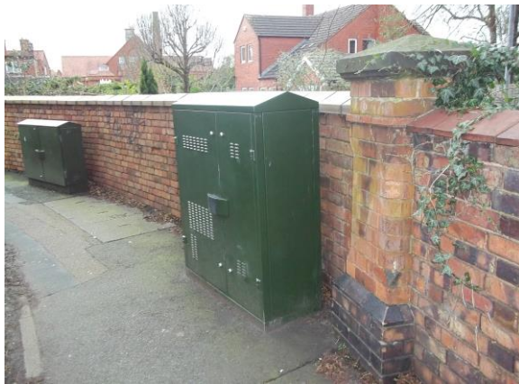
Figure 5: Unsympathetic telecommunications boxes adjacent historic wall
