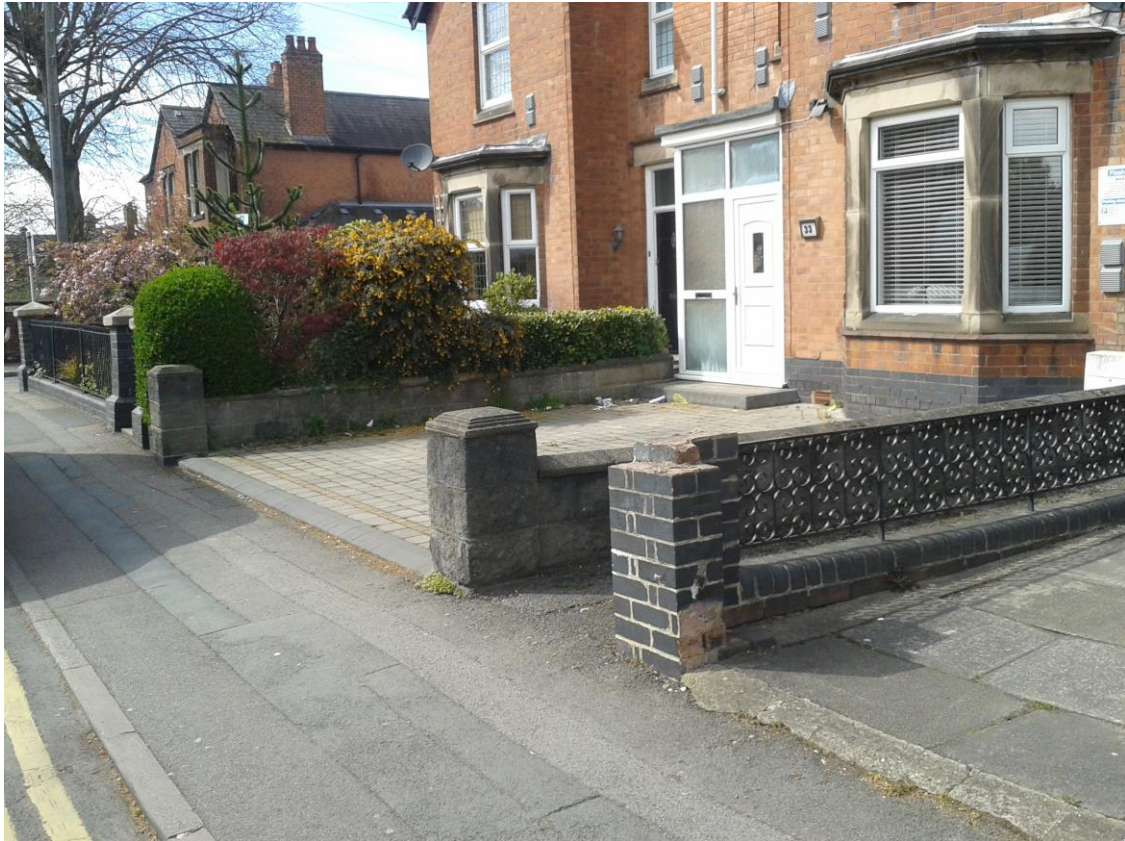
Figure 9: Removal of boundary treatment for parking and inconsistent palette of materials from the original which is shown as a plinth and railings further along the street.
