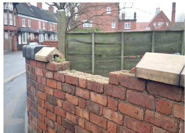
Figure 6: Coping and brickwork missing from wall
