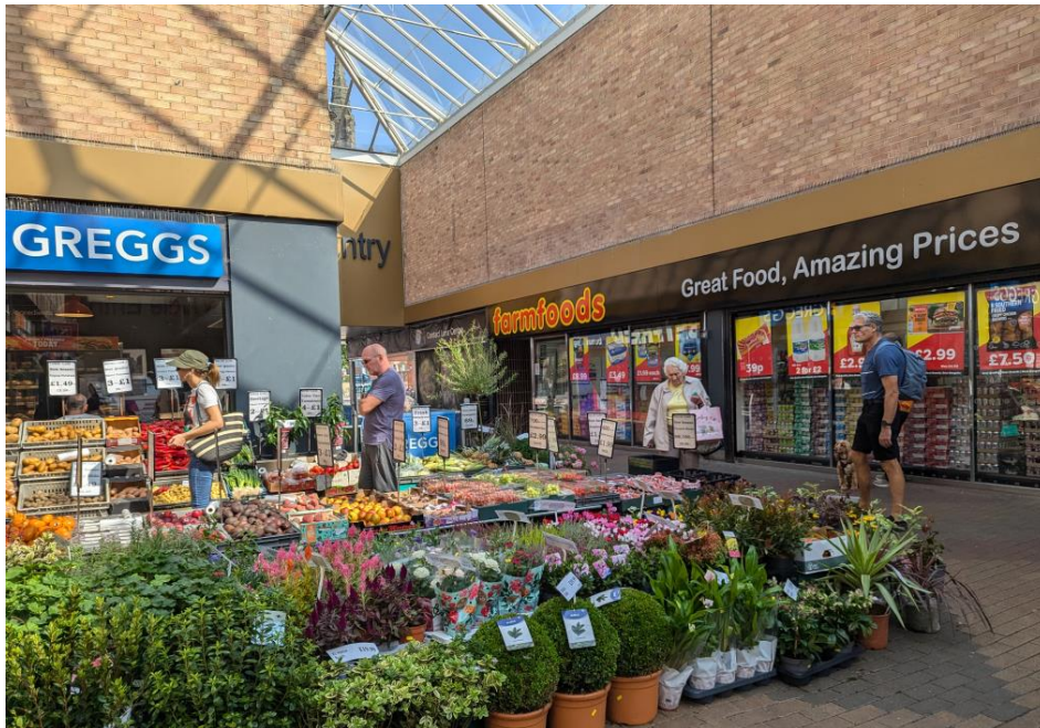
Current retail offer in Middle Entry, showing the glazed roof which will be removed under approved plans.
