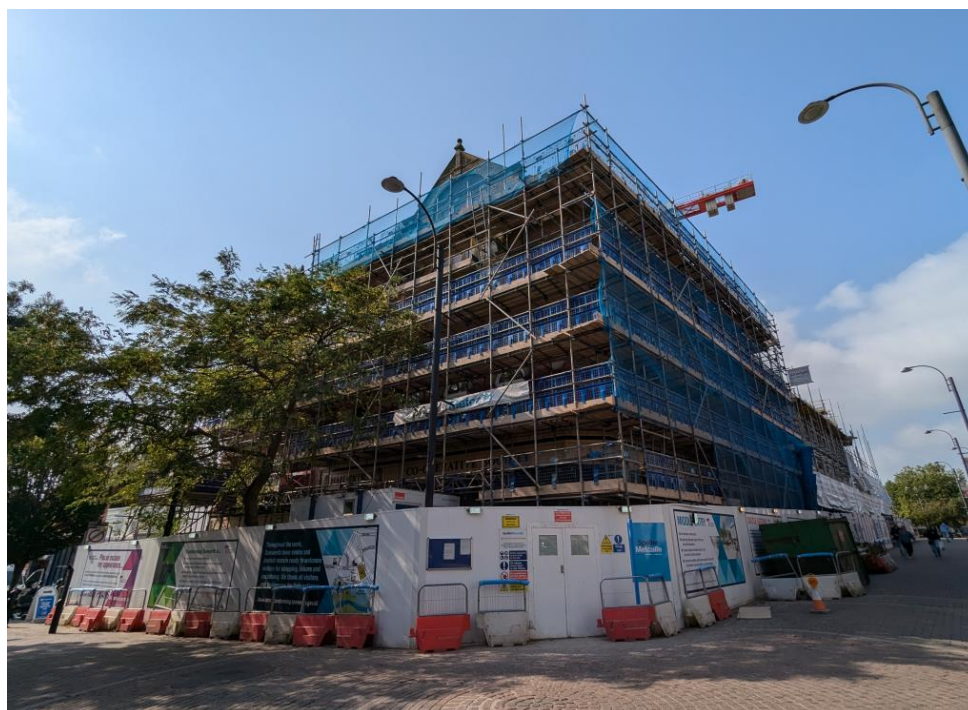
New Enterprise Hub under development, Coleshill (September 2024)
